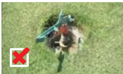
Exposed irrigation head
