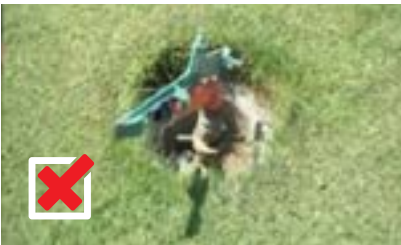
Exposed irrigation head
