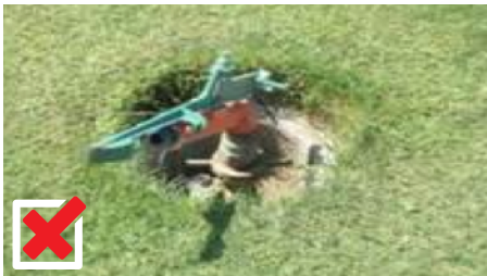
Exposed irrigation head
