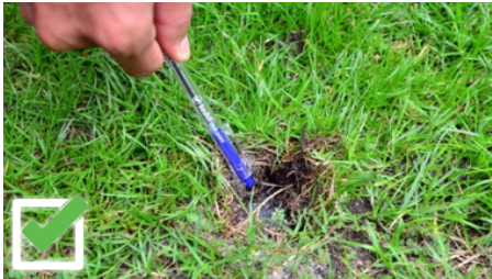
Concealed sprinkler head
